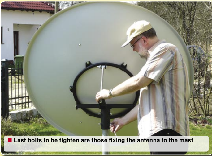
■ We used an LNB we had in the drawer, so the original feedhorn and its support were not needed
