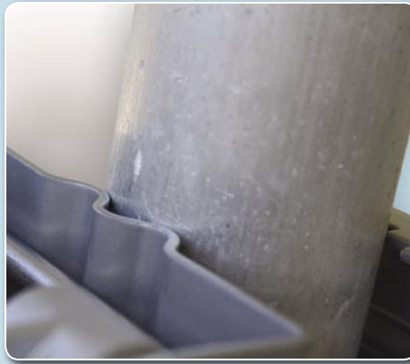
Mark for aligning the motor on the mast to the South
